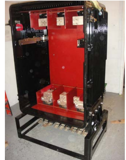
Installing submersible equipment
